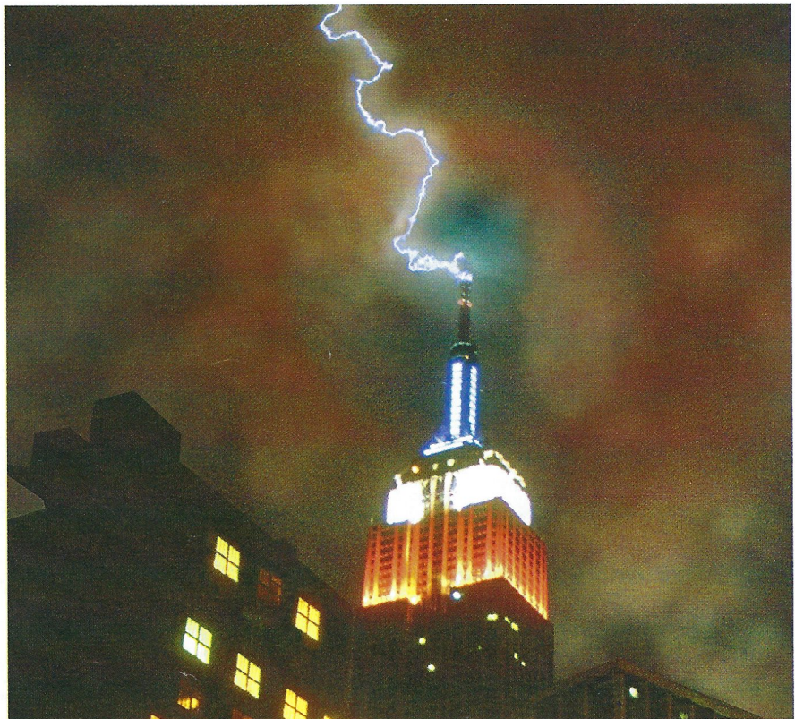
Figure 7 Lightning strikes the lightning rod rather than the building, because the lightning rod is the tallest point on the building.
